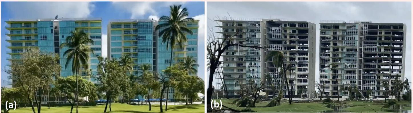
Fig. SB4.2. (a) Before and (b) after view of high-rise buildings and surrounding vegetation highlighting the severe wind impacts from Hurricane Otis in Acapulco, Mexico. (Photo credit: Parvez 2023.)
